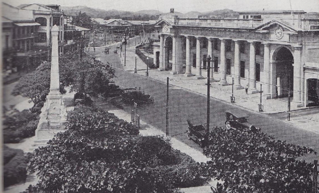
PANAMA RAILROAD STATION, PANAMA CITY
