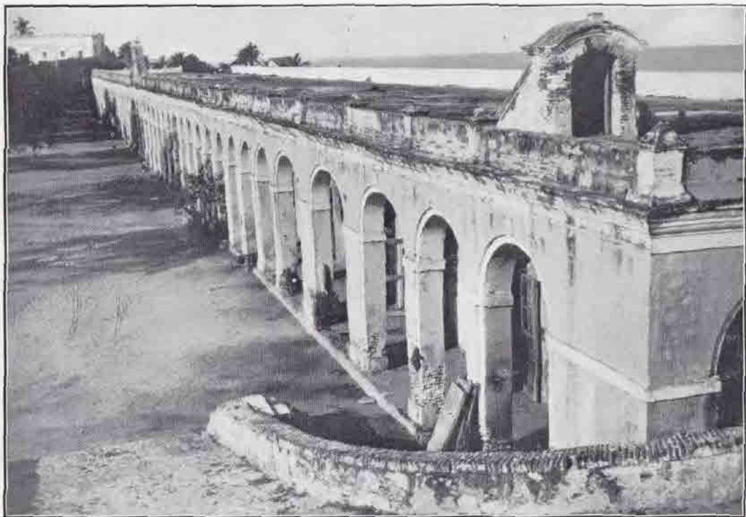
CARTAGENA—Part of the City walls known as "Las Bovedas"; the walls at this point are over 80 feet in width. In the time of the Spaniards the archways were used as prisons, and the top of the walls as parade grounds. The building in the background is the Hospital of Santa Clara.
